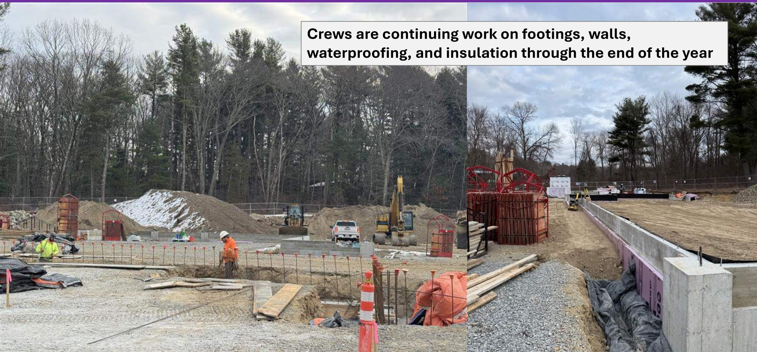
**Crews are continuing work on footings, walls, waterproofing, and insulation through the end of the year**
