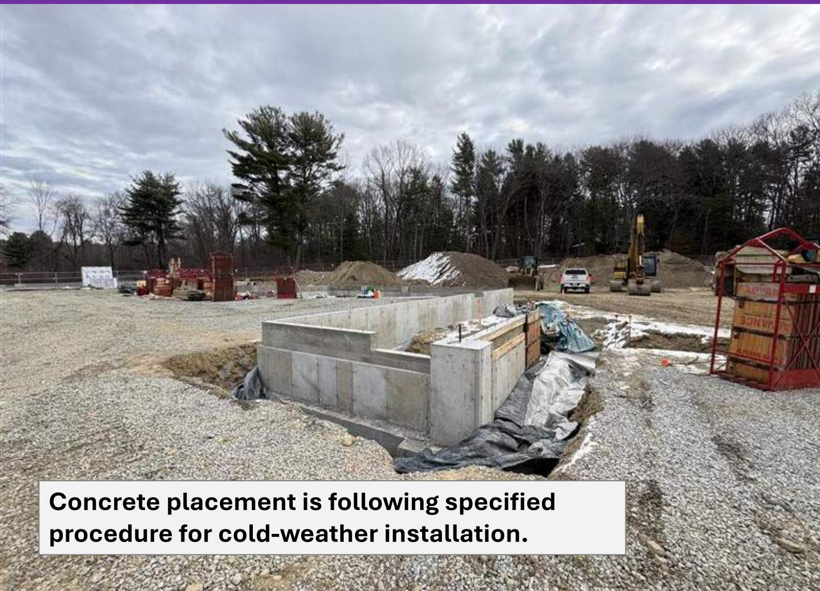
**Concrete placement is following specified procedure for cold-weather installation.**
