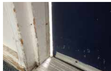
Exterior Doorway Condition
