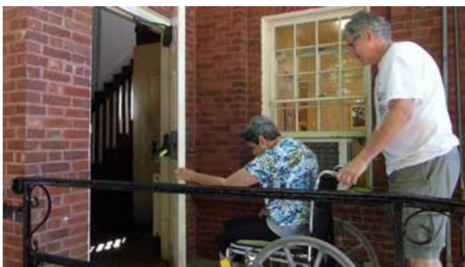
The only ADA-compliant entrance is not ideal.
